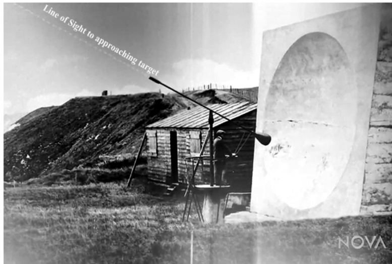
Figure 7. An acoustic mirror similar to the one at Kilnsea (PBS Learning Media)
