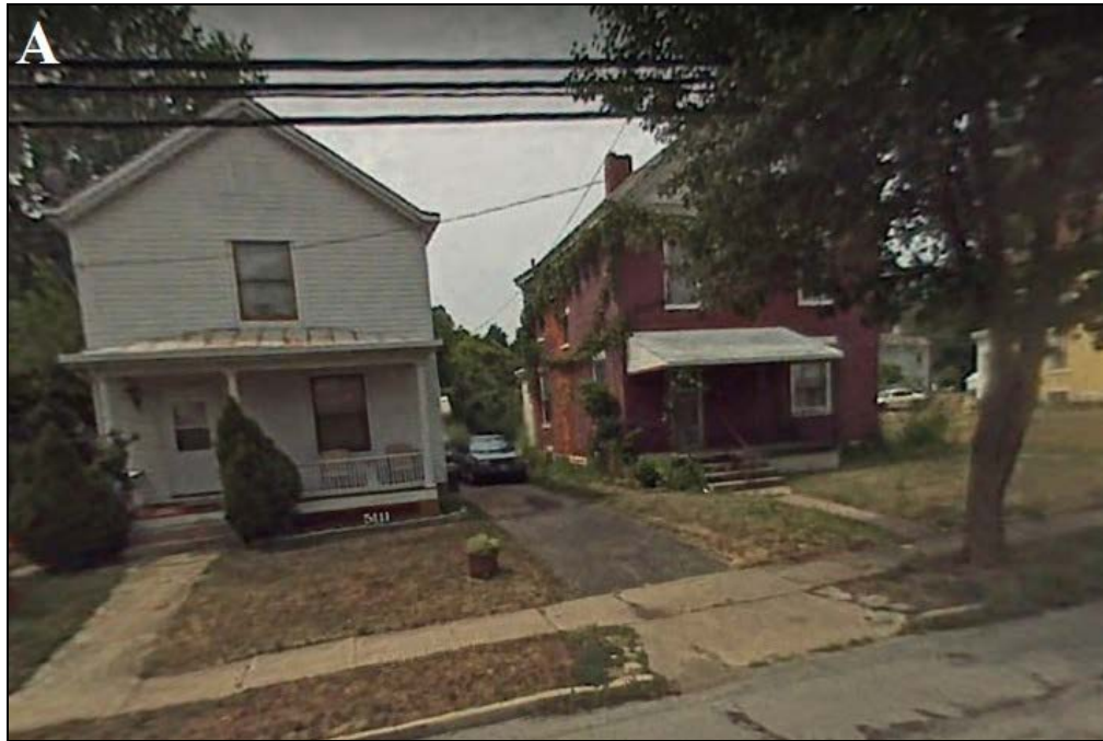
Figure 3. Kenwood Road. (A) Disinvested Houses, 2007. (B) Vacant Lot and Façade Improvements, 2016.
