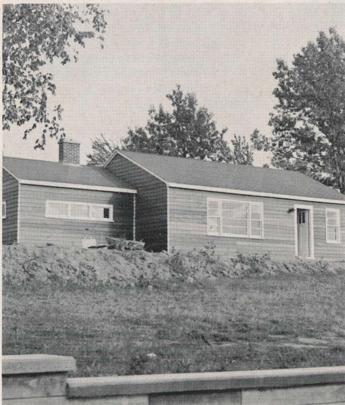
The new heating, ventilating, and air conditioning building constructed this summer by Prof. Kruger, William Azman, and Otto Woike.
