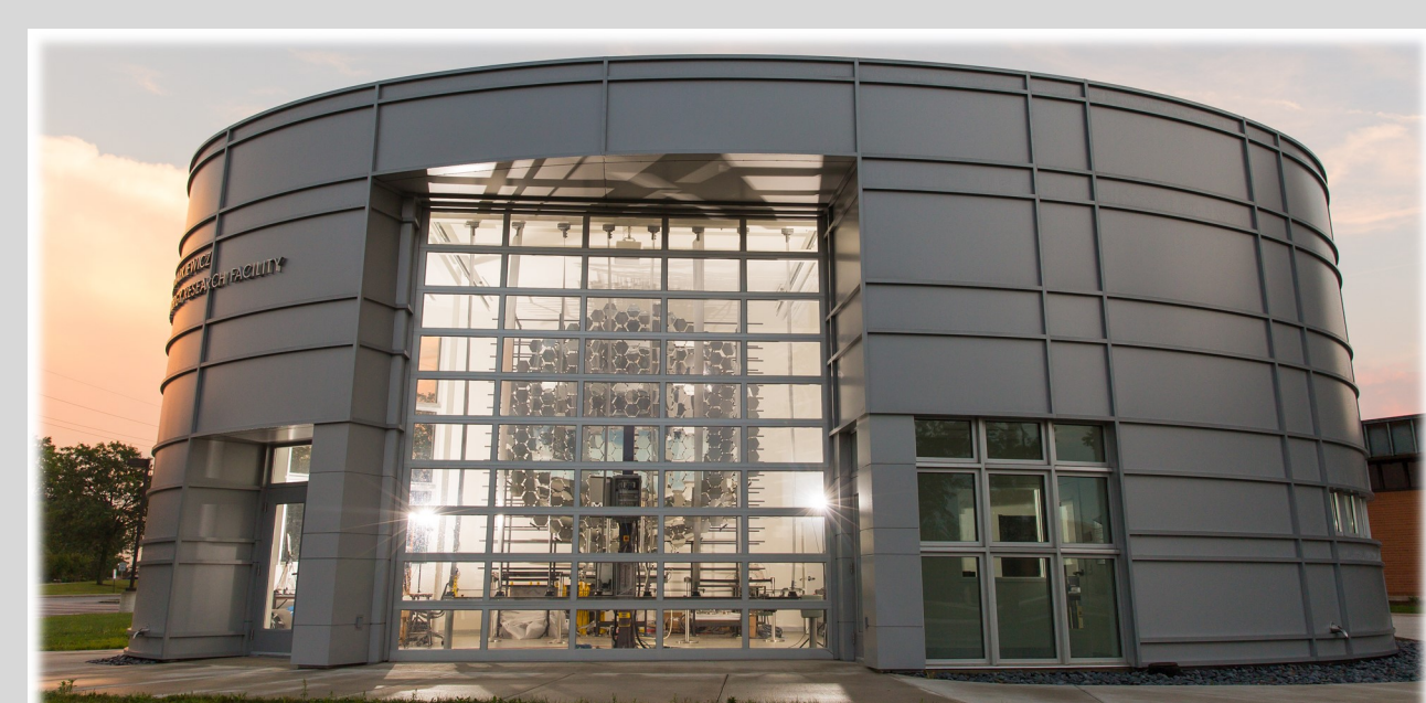
Figure 1: James S. Markiewicz Solar Energy Research Facility
